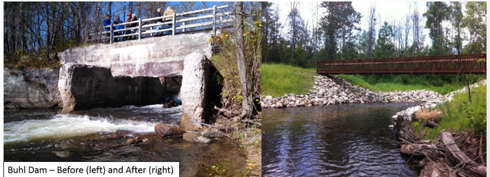
Buhl Dam – Before (left) and After (right)
