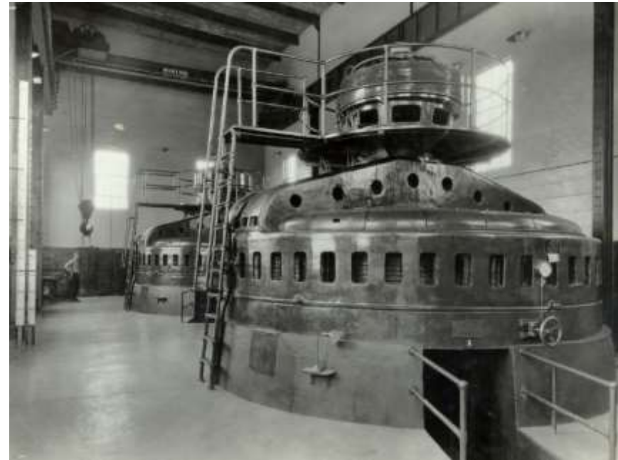
Generating units at Mio Dam
