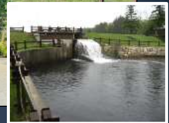
Song of the Morning Dam Removal Project Pigeon River Ribbon Cutting Celebration – Aug. 31, 2016
