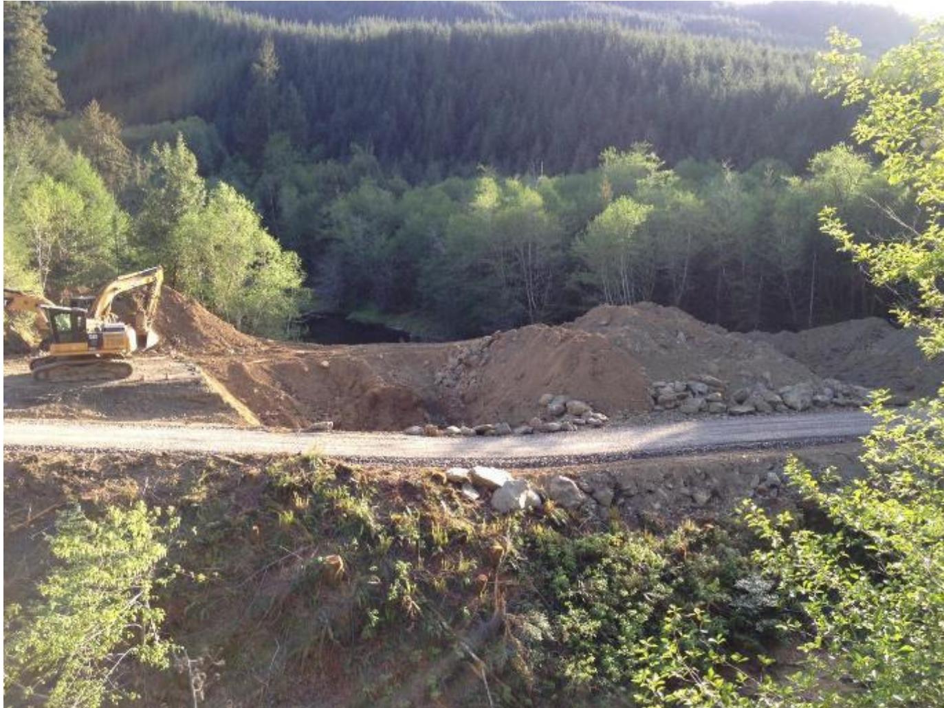
Bridge #4 dig holes in fill to bedrock
