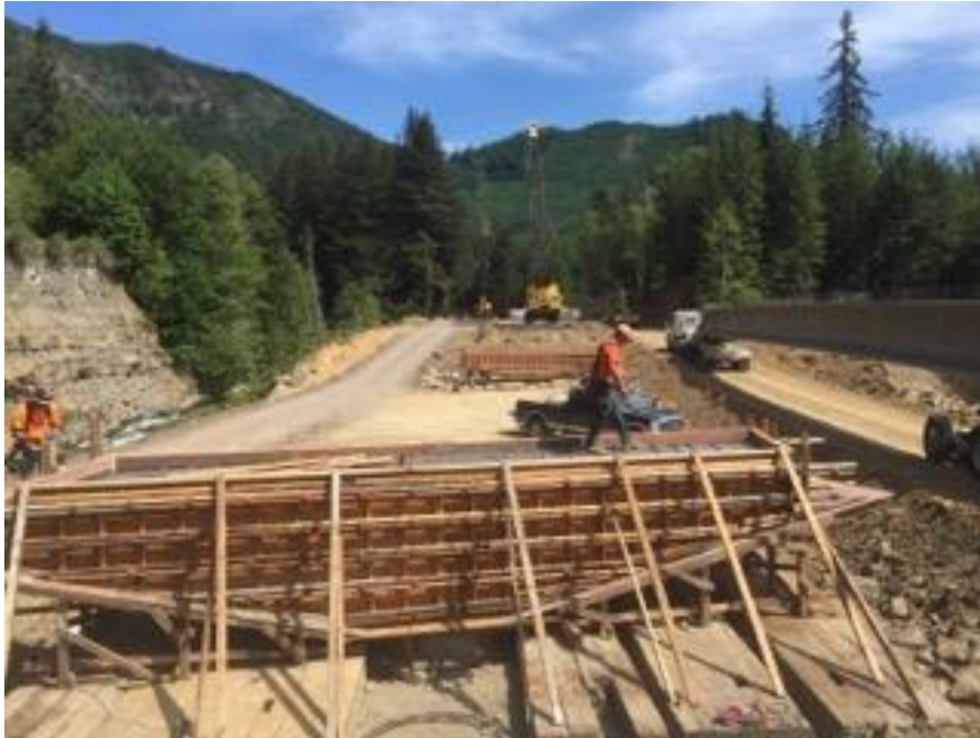
Bridge #4 Constructing hammerheads.
