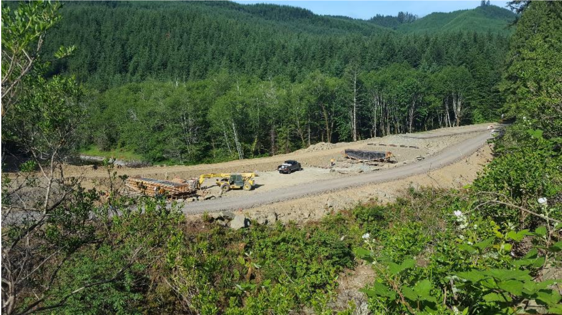
Bridge #4 Constructing hammerheads.
