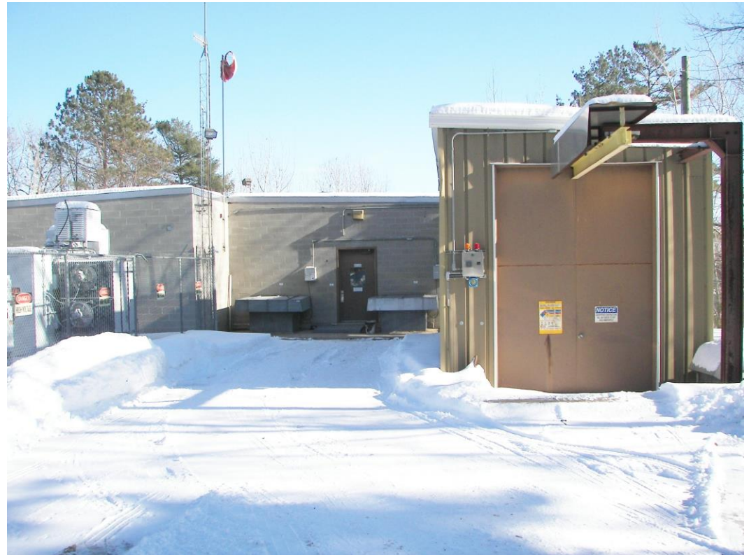
Bay Pumping Station
