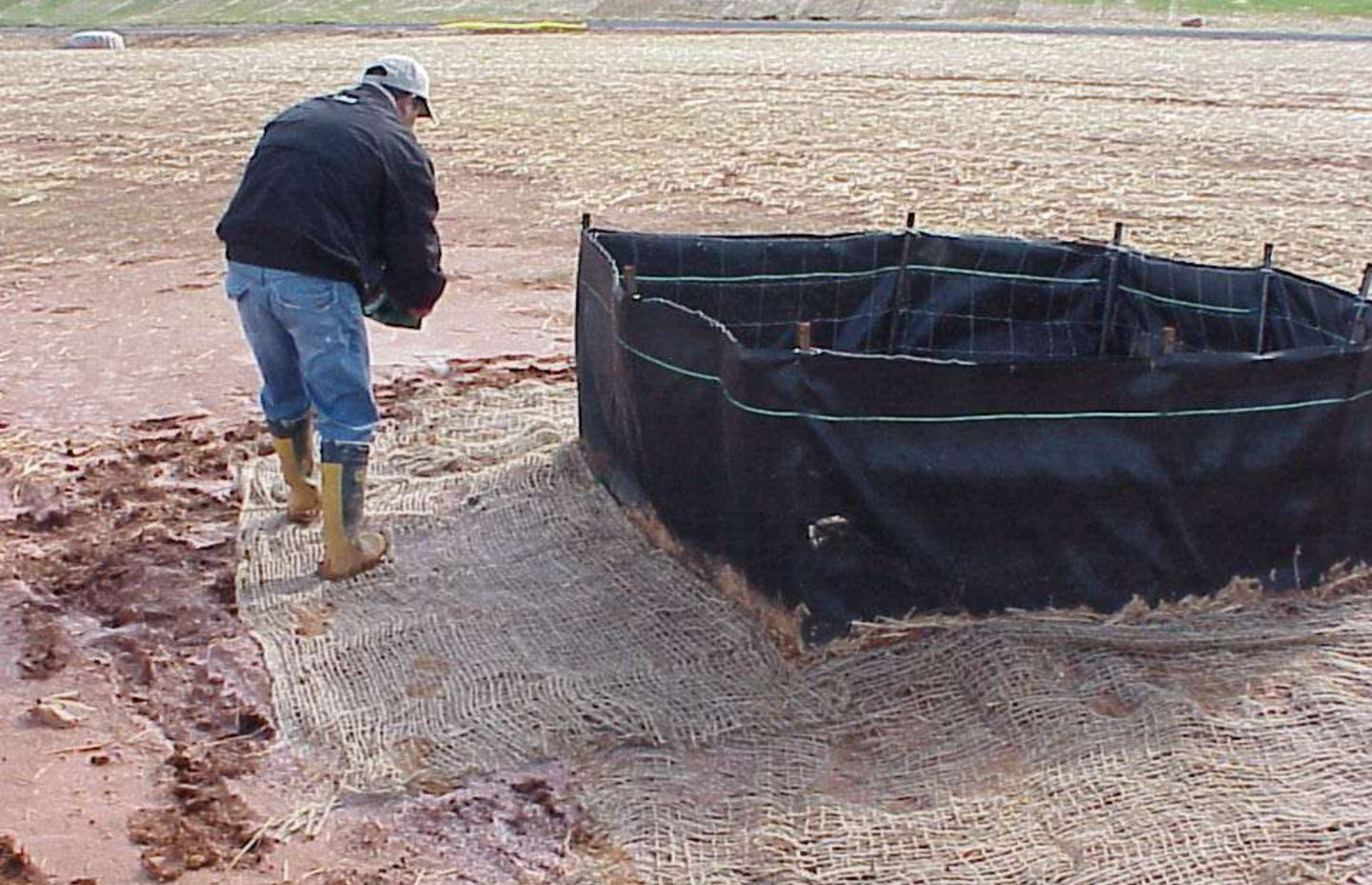
Apply jute matting with the correct soil specific polymer to reduce soil movement at the BMP
