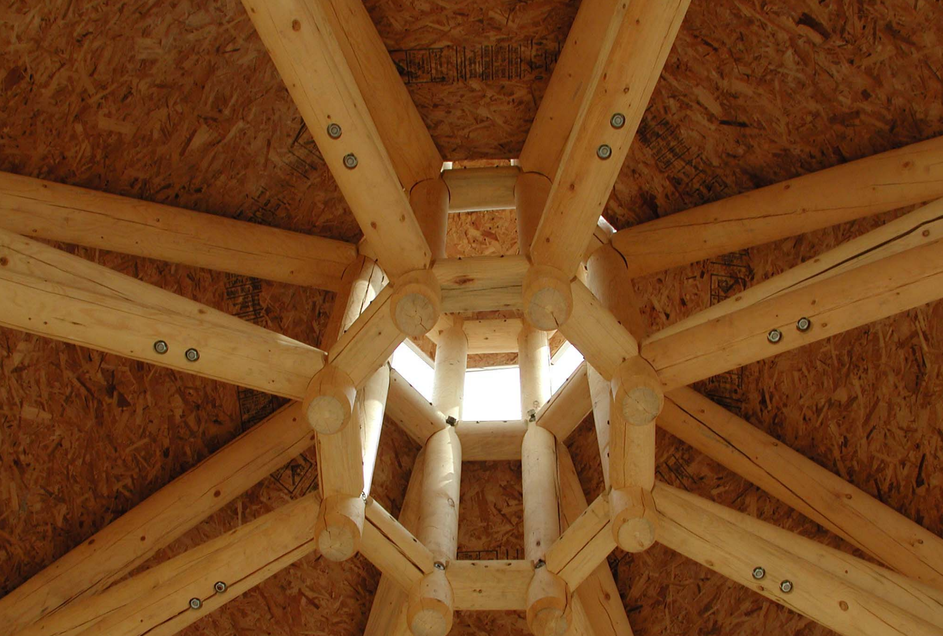
Turned logs Coped ends
