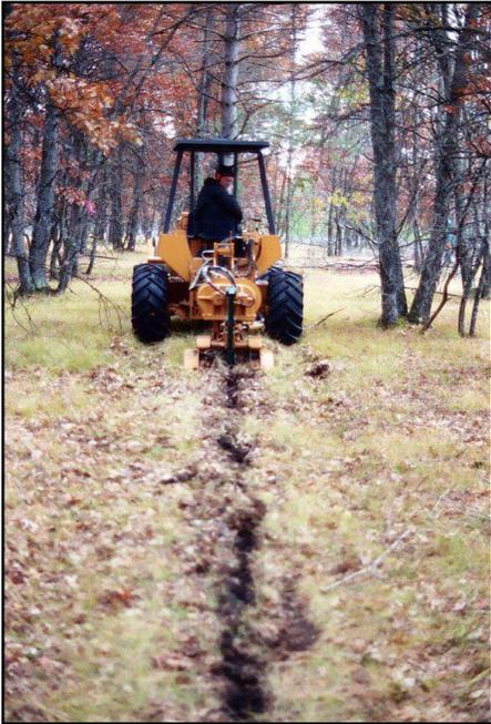
**Vibratory Plowing** (Figure 19): Many miles of oak wilt areas in Michigan have been treated with a vibratory plow pulled behind a large tractor, following the perimeter line delineated around the epicenter. The plow has a blade that slices into the ground, at least five feet deep, facilitated by a powerful vibration action. Plowing must be at least five feet deep to ensure the oak roots are severed. Vibratory plowing should be done during the dormant season.
