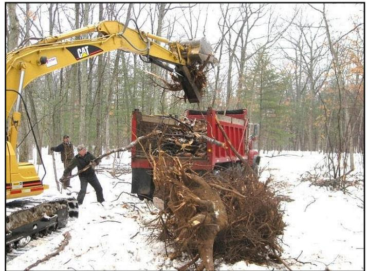
Figure 21. Stump-pulling and chipping.
